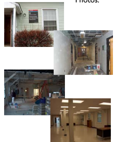
Service Center Renovation Photos:
