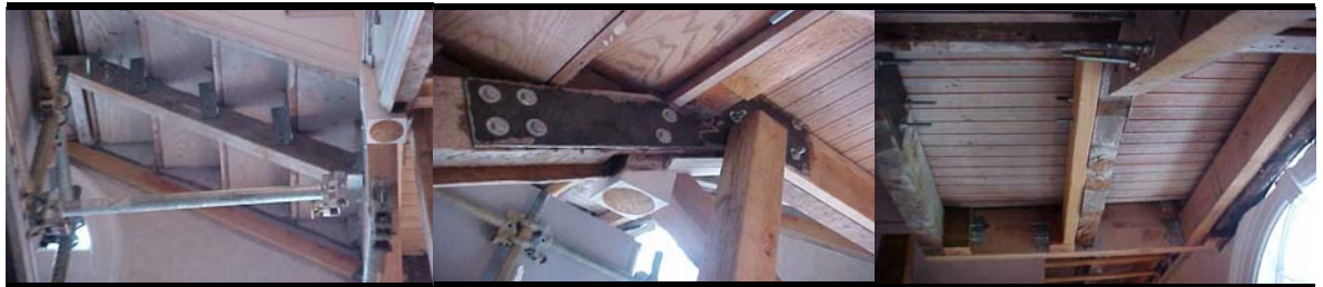
Shoring Up Stairs
