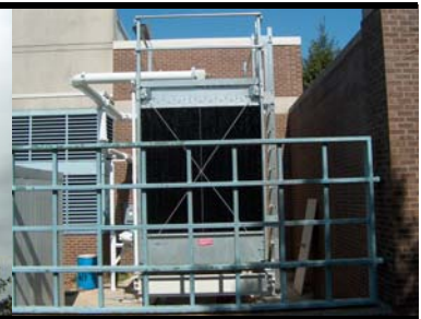
New Tower in Place
