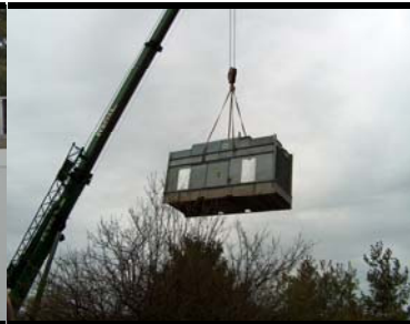
Removal of Existing Tower
