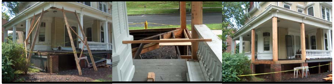
New floor joists, footings & columns
