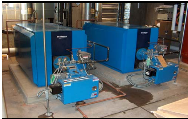
Completed Project: New Boilers
