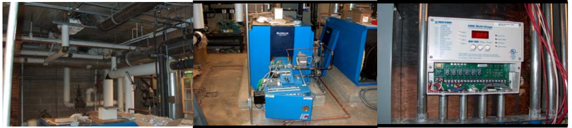
New Ductwork & Piping
