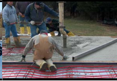
Installation of New Slab
